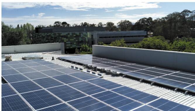
Silver cell solar panel installation on the Anthony Low Building, ANU.
