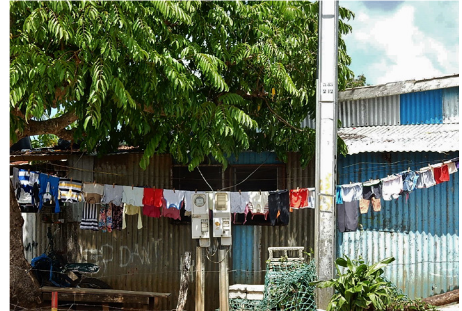
Domestic meets public with a washing line set up around power meters and an electricity pole in Port-Villa, Vanuatu (Photo credit: Michael Coghlan, CC BY-SA 2.0).
