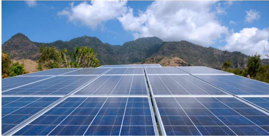
Solar panels in Bali, Indonesia (photo credit: Selamat Made CC BY 2.0).
