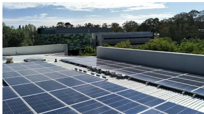
Sliver cell solar panel installation on the Anthony Low Building, ANU.
