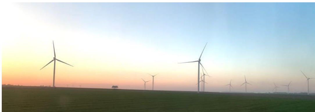
Figure 3: large scale wind generation across the agricultural landscapes of northern Germany.
