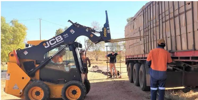
Unloading the hydropanels. (Image: Central Desert Regional Council)
